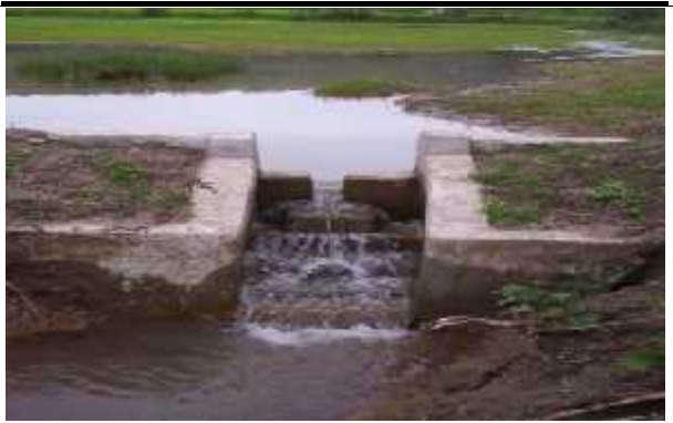
Check dams constructed in cultivable land
