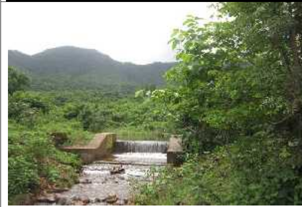
Masonry surplus constructed in drainage line
